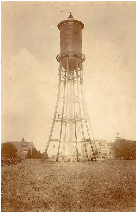
Figure 3.5: The Marston Water Tower This water tower was constructed in 1897. It is 51 meters in height, and rests on an octagonal base. The tank holds approximately 613 Kiloliters
