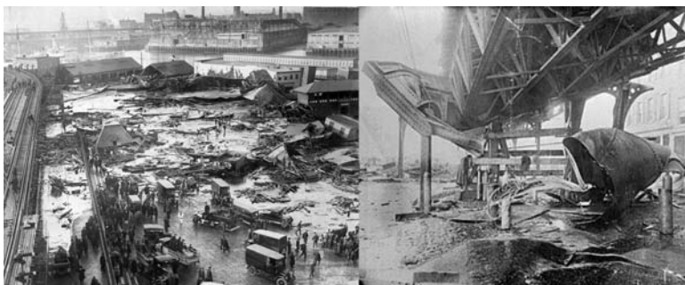
Figure 4.8: Aftermath of the Boston Molasses Disaster. (Left) The remains of the collapsed storage tank are visible next to the light colored warehouse (Right) Damage to the Boston Elevated Railway
